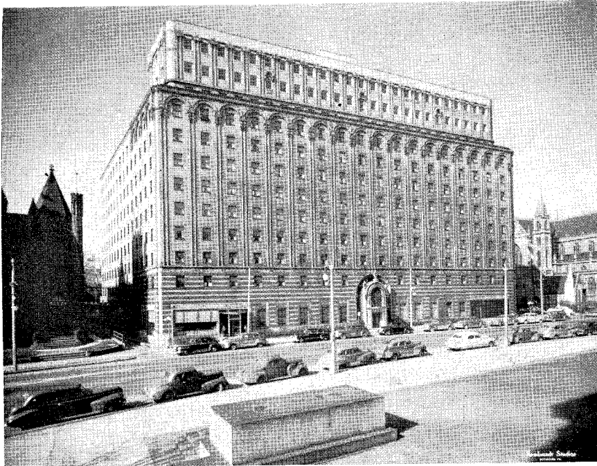
Webster Hall Hotel, Oakland district, Pittsburgh, where the 1950 convention will be held May 1, 2 and 3.
